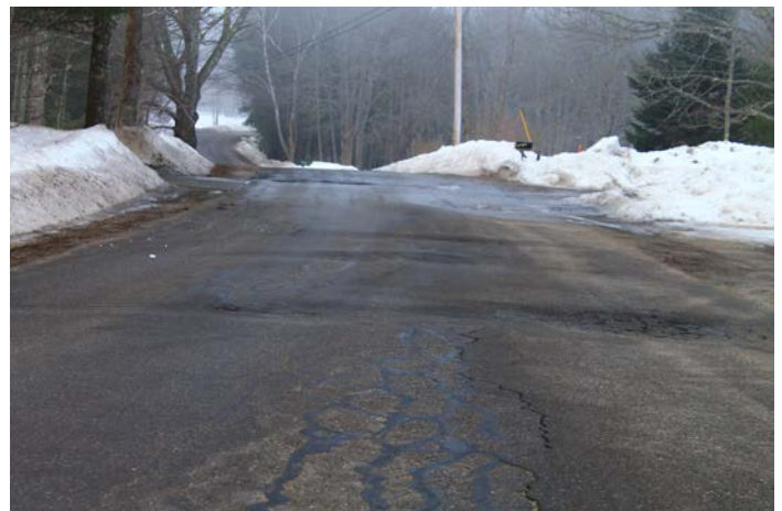
Curtis Road – FY 2018 Road Reconstruction Project. Photo Courtesy Town Staff
